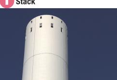
After being treated in the Bag Filter and Denitration Reaction Tower, the exhaust gas is released into the atmosphere through the 85-meter stack. The concentrations of hazardous substances contained in the exhaust gas meet Japan's most stringent environmental standards.
