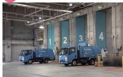
The collected solid waste is dumped into the Waste Pit through the Waste Dump Doors on the Platform. Automatic sliding doors and an air curtain at the entrance to the Platform help prevent odors from escaping the facility.
