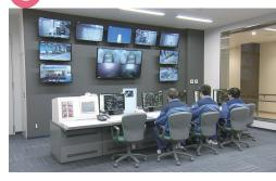
Operation and monitoring of the various processes within the facility are carried out automatically 24 hours a day. The control computer receives a continual flow of information as well as images from surveillance cameras as it monitors the operational status of the various processes within the facility.
