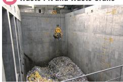
The Waste Pit can hold about a week's worth of solid waste. An automated Waste Crane feeds the accumulated waste into the Incinerator, The Waste Crane can hold up to five metric tons of waste at one time.
