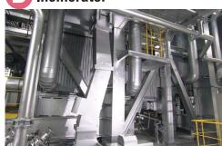
The incinerator contains two furnaces that can incinerate 114 metric tons of solid waste per day. The waste is completely burned in these furnaces at a minimum temperature of 850 degrees Celsius. This high temperature suppresses the generation of dioxins and other hazardous substances.
