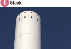
After being treated in the Bag Filter and Denitration Reaction Tower, the exhaust gas is released into the atmosphere through the 85-meter stack. The concentrations of hazardous substances contained in the exhaust gas meet Japan's most stringent environmental standards.
