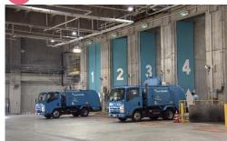
The collected solid waste is dumped into the Waste Pit through the Waste Dump Doors on the Platform. Automatic sliding doors and an air curtain at the entrance to the Platform help prevent odors from escaping the facility.
