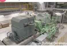
The heat generated by incineration of the waste is fed to the boiler. There, water is heated to generate high-pressure steam that is used to spin the blades of the steam turbine and drive the generator to produce electricity. The rated power generation capacity is 5,190 kW.
