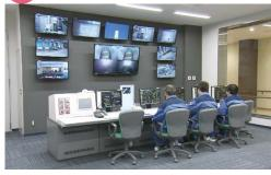
Operation and monitoring of the various processes within the facility are carried out automatically 24 hours a day. The control computer receives a continual flow of information as well as images from surveillance cameras as it monitors the operational status of the various processes within the facility.
