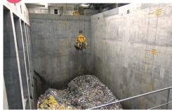
The Waste Pit can hold about a week's worth of solid waste. An automated Waste Crane feeds the accumulated waste into the Incinerator. The Waste Crane can hold up to five metric tons of waste at one time.
