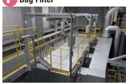
Slaked lime and activated carbon are sprayed into the exhaust gas passing through the Bag Filter. The ensuing chemical reactions ensure that dioxins, hydrogen chloride, sulfur oxides, mercury, and any other hazardous substances are collected by the filter cloth in the Bag Filter.
