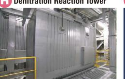
The fly ash collected in the Bag Filter is circulated through In the Denitration Reaction Tower, nitrogen oxides are removed as they are decomposed into environmentally harmless nitrogen and water. This decomposition is achieved by blowing vaporized aqueous ammonia into the exhaust gas and passing the mixture through a catalyst.
